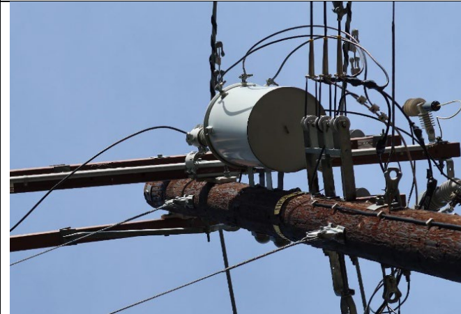
IA1mg2: View showing primary bushing avian protection open
