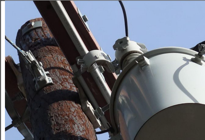
IA1mg1: View showing primary bushing avian protection open
