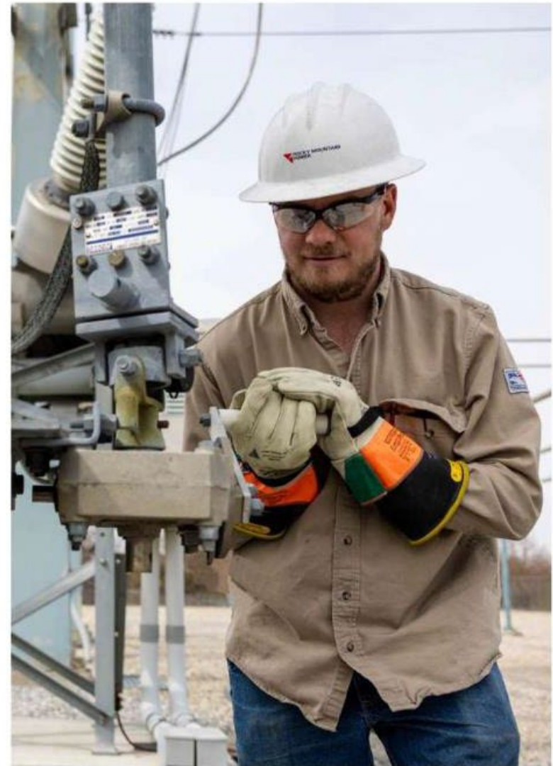
Safer switching equipment is an example of engineering advances.
