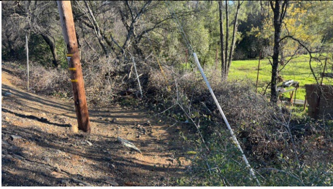
Photo 3: Photo of the tan oak wood and slash debris, accumulated along the outer ring of the structure Pole ID 100380208.
