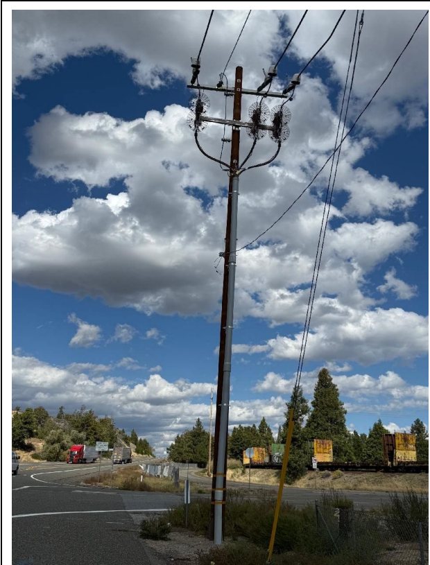
G1mg1: Overall Structure
