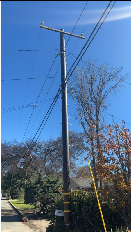
G1mg1: Overall Structure
