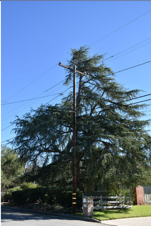
IA1Img1: Overall Structure
