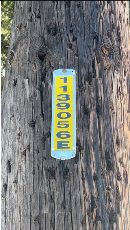
IA1Img2: Structure ID
