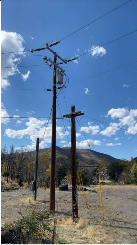
IA1Img1: No covered conductor installed heading northwest of Pole 06246009.135501.
