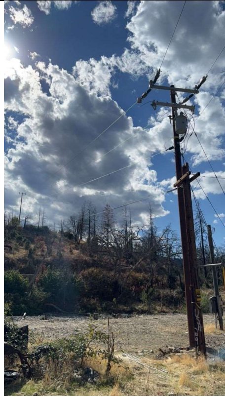
IA1Img2: No covered conductor installed heading northwest of Pole 06246009.135501.
