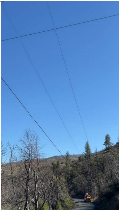
IA1Img3: No covered conductor installed on the east side span along Klamath River Road to next pole with Pole ID 06246009.133400.
