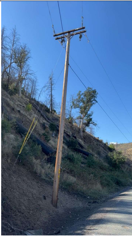
IA1Img4: The next pole, Pole ID 06246009.133400 with no covered conductor installed.
