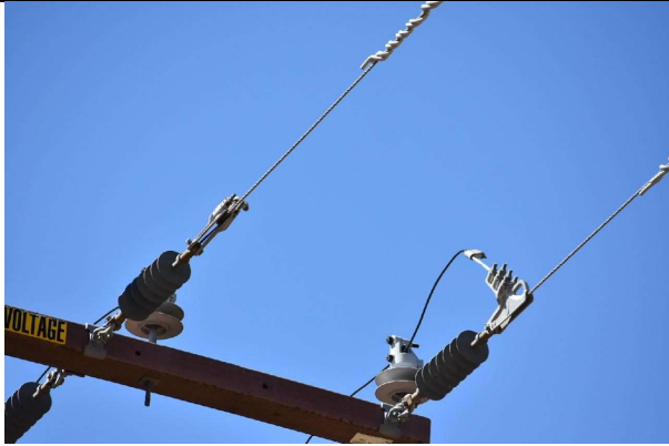
IA1Img3: No Covered Conductor observed
