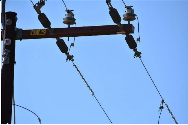
IA1Img4: No Covered Conductor observed
