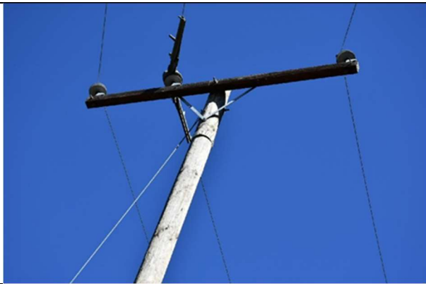
IA1Img4: View of bare conductor
