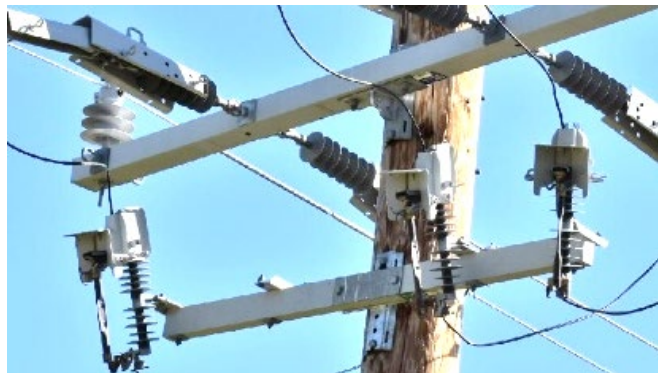
IA11mg2: Three solid blade disconnects were installed (detailed view).
