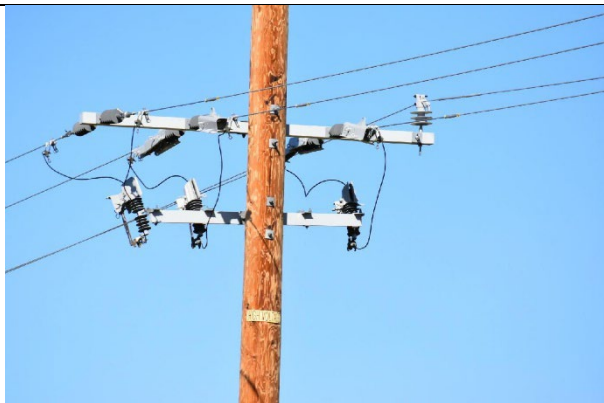
IA11mg1: Three solid blade disconnects were installed.
