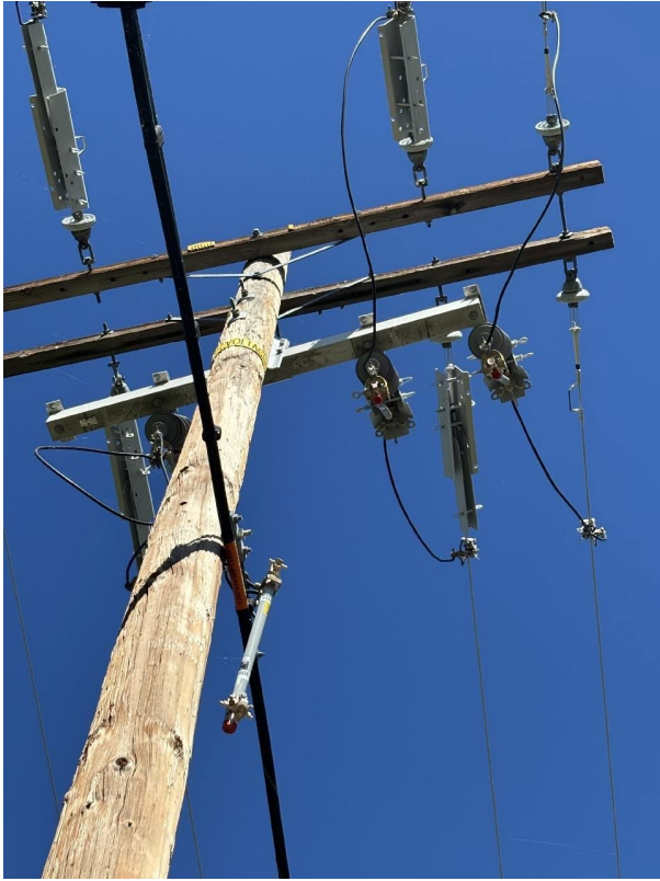
Item1IA1Img1: One CAL FIRE-approved non expulsion fuse not installed in the cutout.
