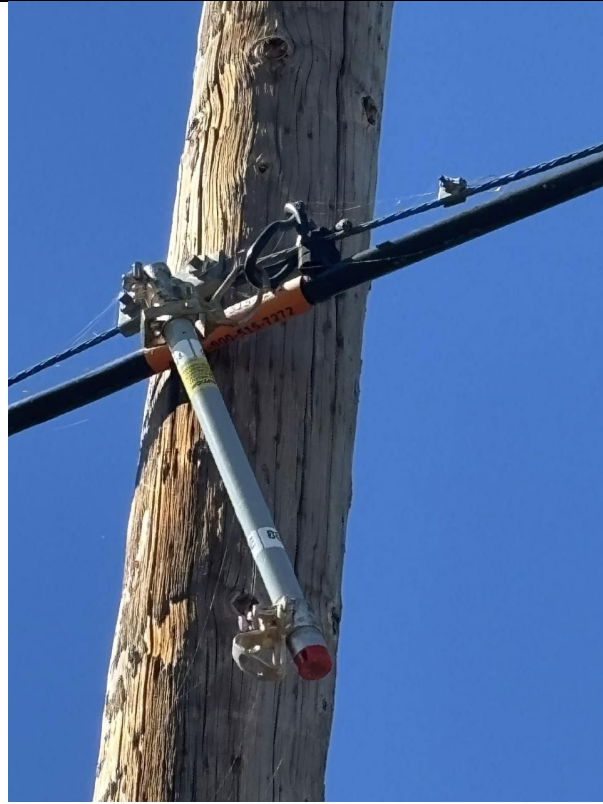
Item1IA1Img2: One CAL FIRE-approved non expulsion fuse hanging from the pole.
