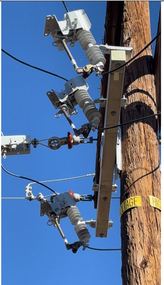
IA1Img1: Solid blade disconnects installed
