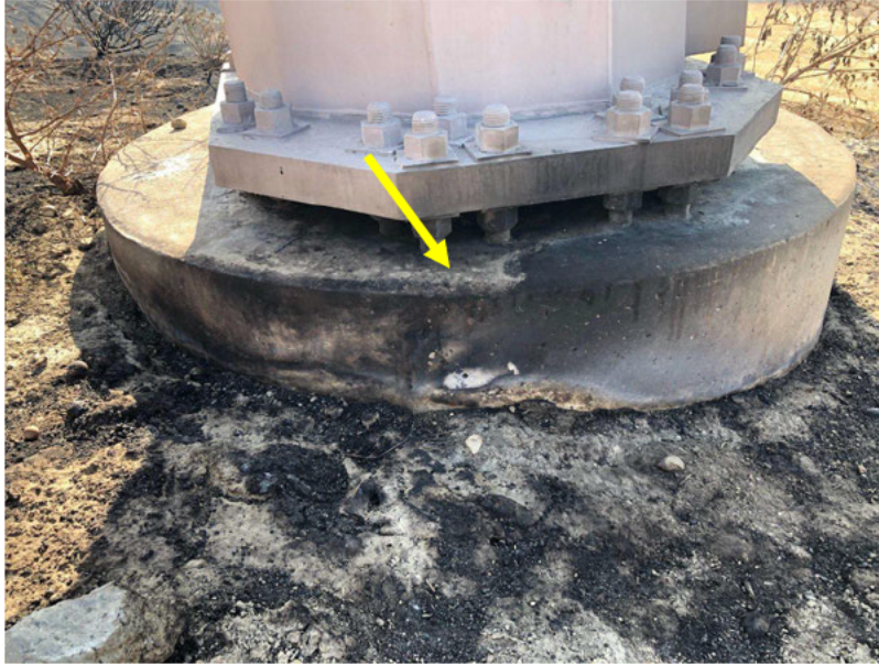
Figure 6: LAFD photograph showing evidence of unusual burning on one of the footings on Tower M2-T4.
