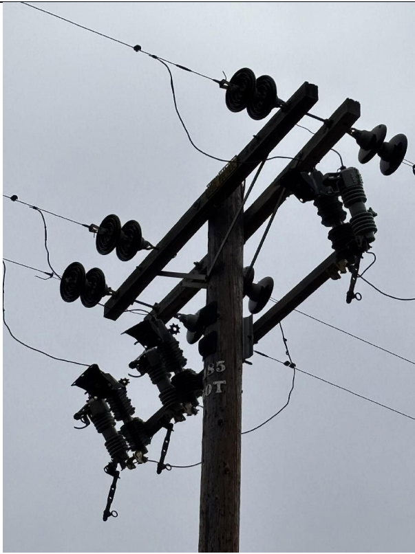
Item1IA1Img1: CalFire-exempt fuses not installed in the cutouts
