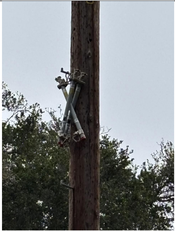
Item1IA1Img2: CalFire-exempt fuses hanging from the pole
