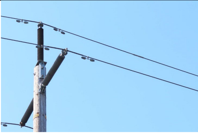
Item1IA1mg3: A splice with no shunt on span between 000/004 and 000/005.
