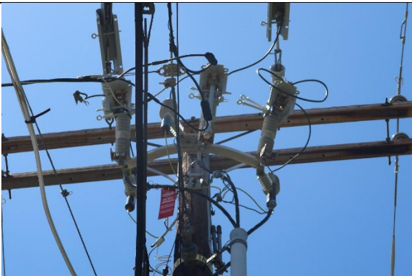
Item1IA1Img1: Two of three fuses not installed in the cutouts.
