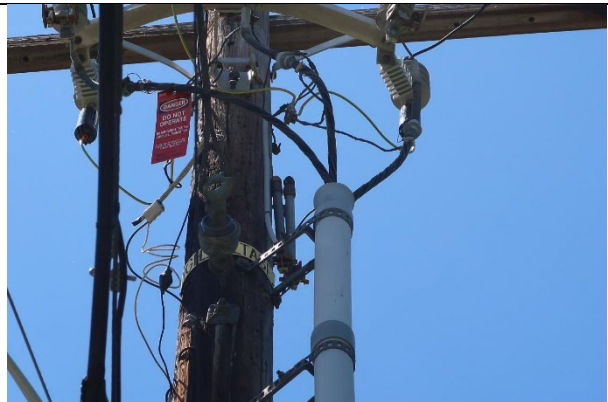
Item1IA1Img2: Two fuses hanging from the pole.
