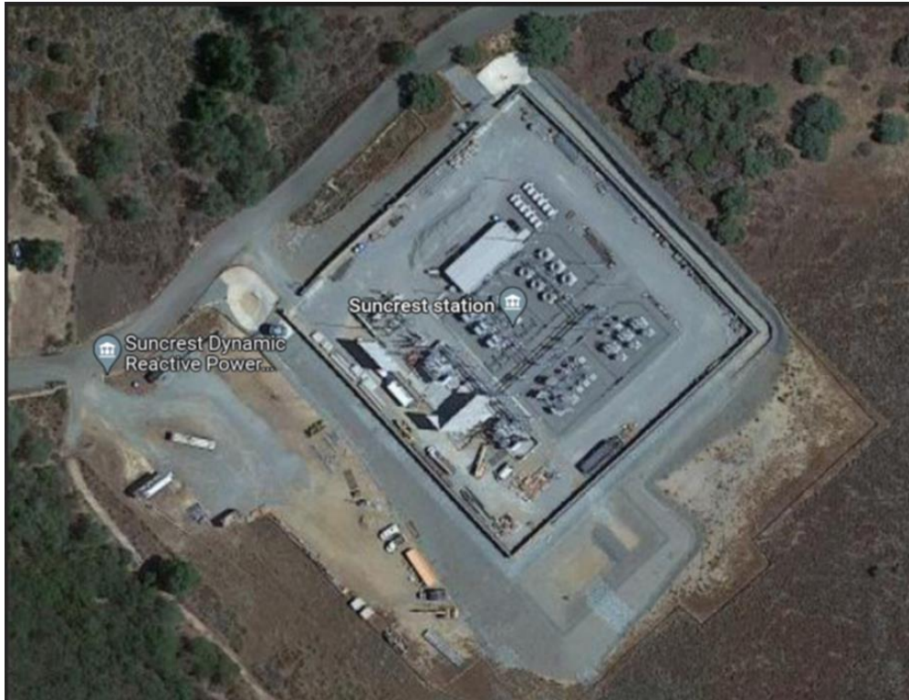
Figure HWT 4-2. Overhead Close-up of Suncrest SVC
