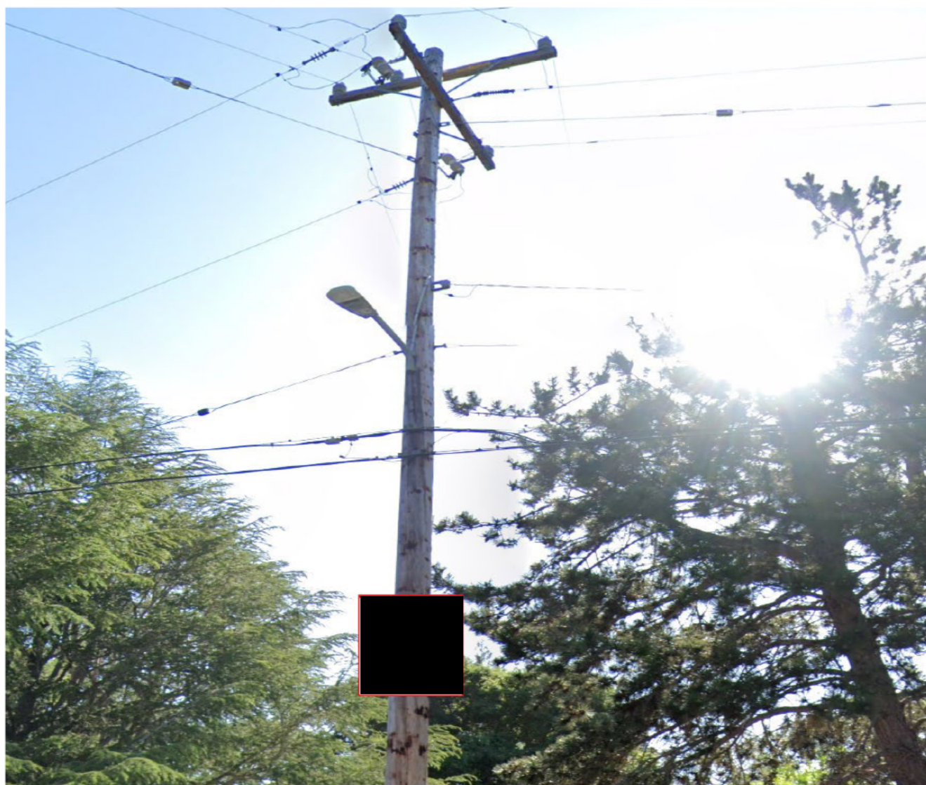
Image 1: Correct structure (pole ID [REDACTED]) with completed replacement Non-Exempt Expulsion Fuse with Solid Blades.
