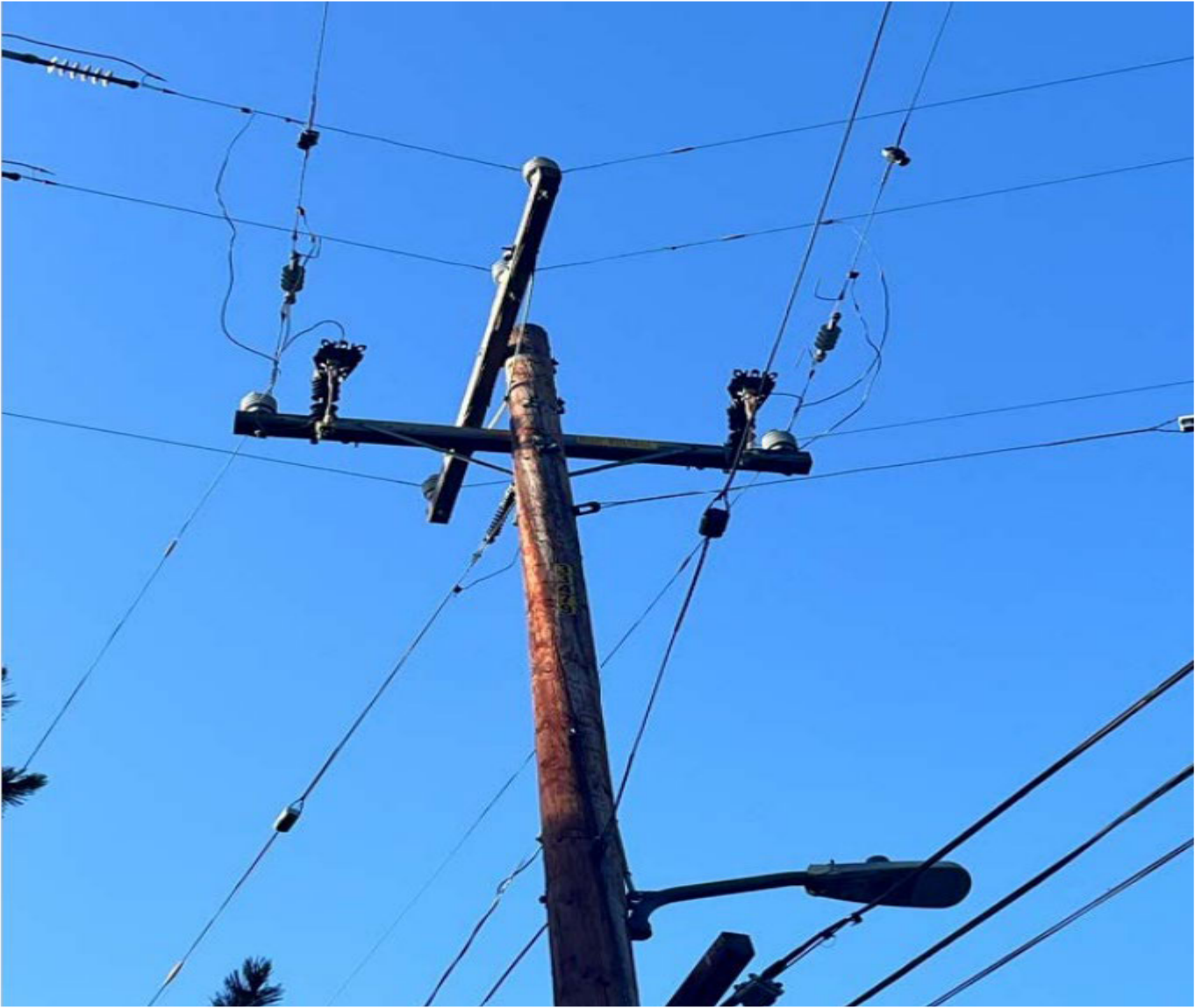
Image 2: Zoomed in view of pole ID [REDACTED] with completed replacement Non-Exempt Expulsion Fuse with Solid Blades.
