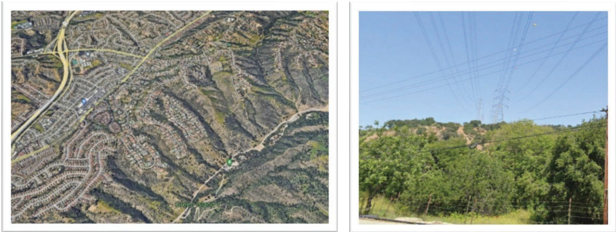
Figure SCE 5-11: Example of a CEFC with Topographical Overview (Left) and Example of Vegetation in Canyon (Right)
