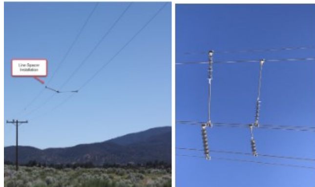
Figure SCE 8-05: A Line Spacer Installed on a Long Span to Mitigate Wire-to-Wire Contact (Left), Close Up Line Spacer View (Right)
