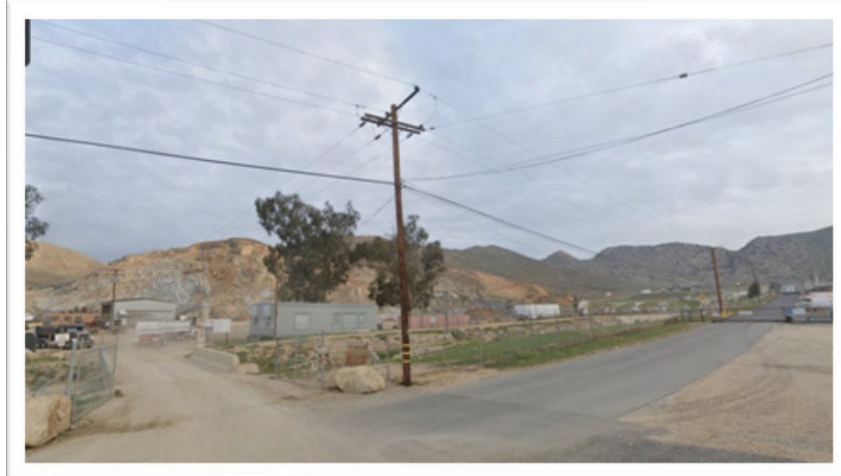
Figure SCE 5-17: Photo of Location Confirms Need to Convert Designation from SRA to HCA
