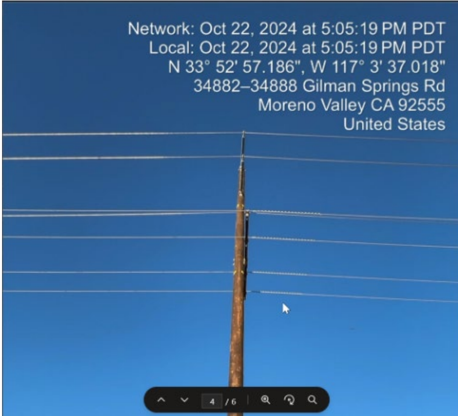
Photo 4 – Covered Conductor Installation Structure ID 4491271E
