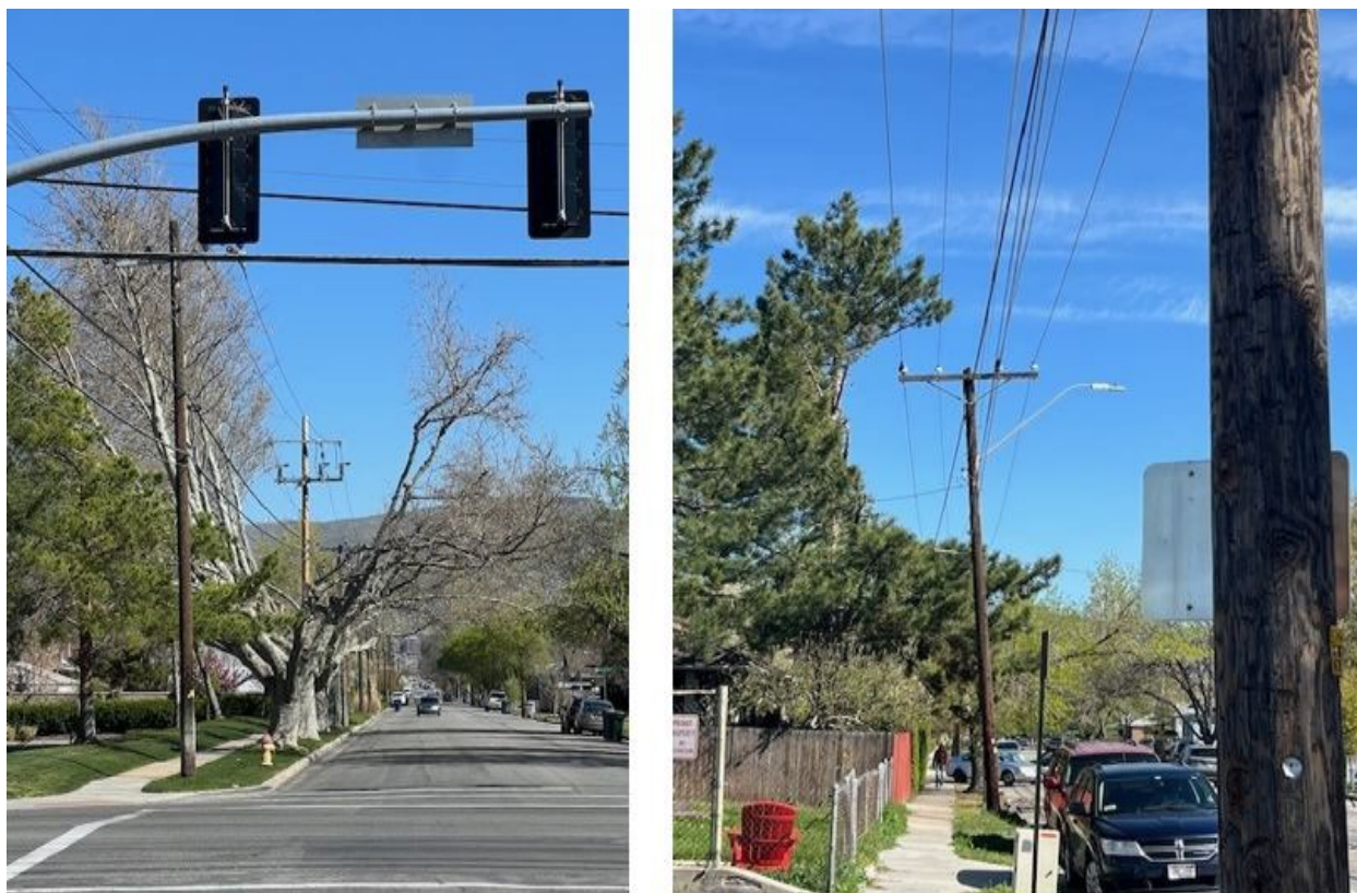
Figure 3.3 “V” or “L” shapes can develop from crown reductions on trees growing in close proximity to power lines. The ultimate objective is to train the tree up and away from the conductor whenever possible, so the facility is cleared while minimizing health risks to the tree.
