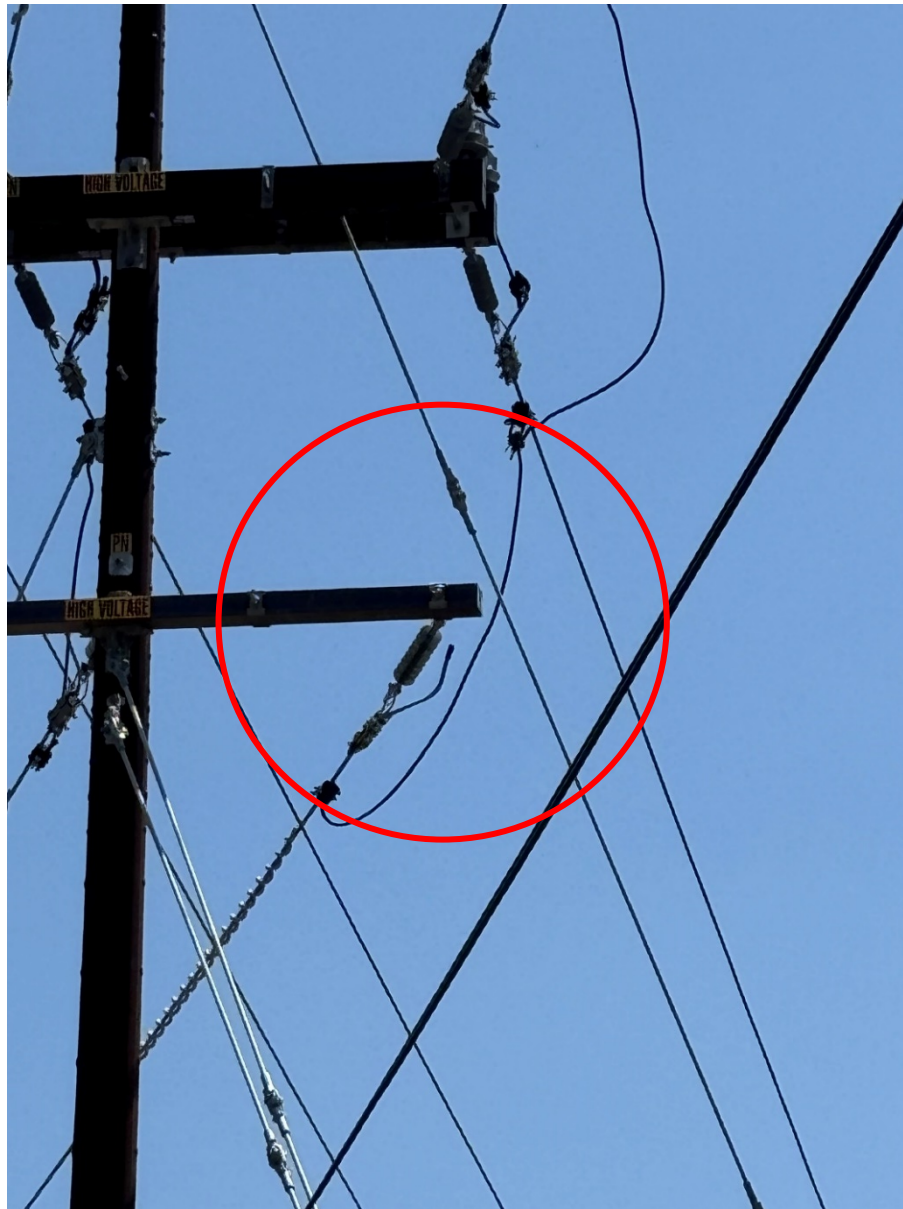
Figure 6 - Image captured on 6/24/2025 by SDG&E construction team after modification of facility
