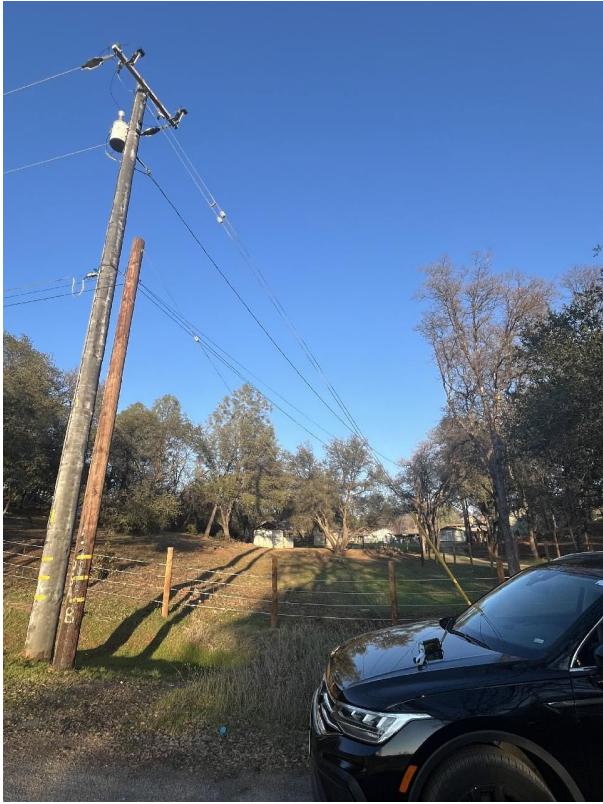
Item1IA1img1: No covered conductor installed east of pole 121530972
