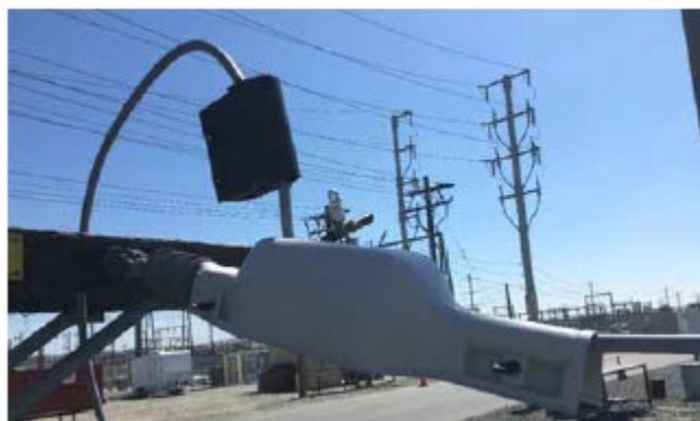
Figure CC 150-3: Connector Cover Installed at Dead-End Tap
