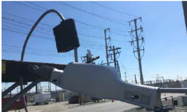
Figure CC 150-3: Connector Cover Installed at Dead-End Tap
