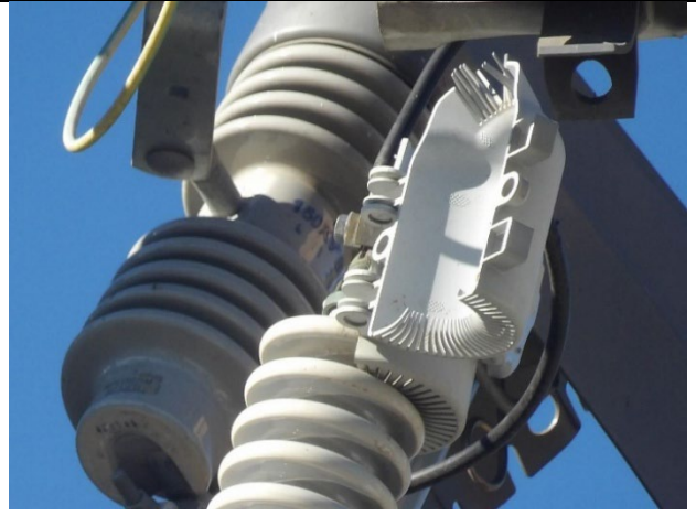
Item1IA1Img2: Close-up view of open wildlife bushing cover.
