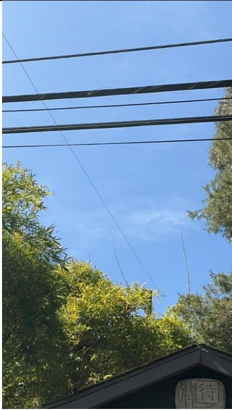
ItemV2: The bamboo culm (left culm) within two feet of the conductor behind the residence.
