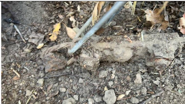
Item1IA1img3: Close up of excavated anchor head below grade.
