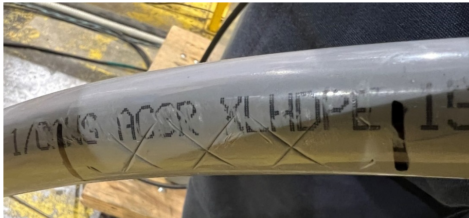
Figure 6-15: Sample 3.2.2 - 35 kV, 1/0 AWG ACSR Condition after Test
