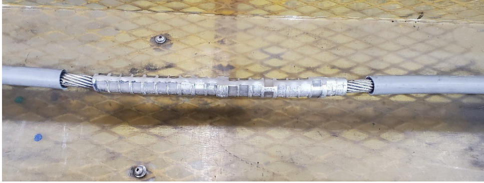
Figure 3-4: [REDACTED] Installed on 22 kV 397.5 kcmil, 19 strands AAC
