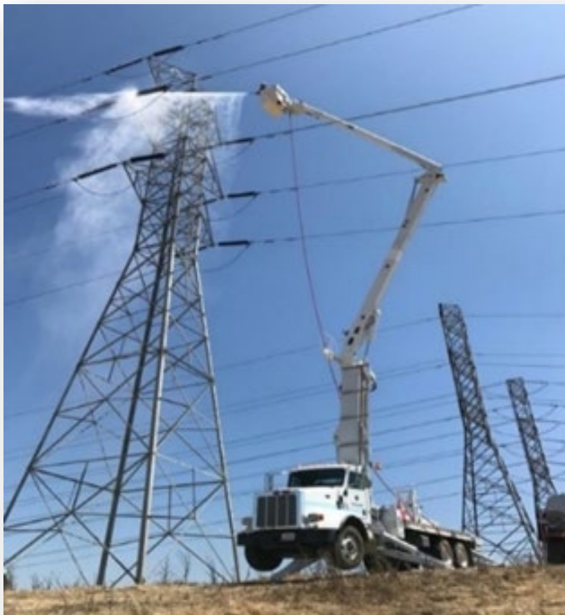
Figure 14 – HHW Line Crew Hot Washing
