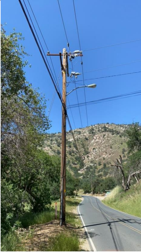
Item7G1mg1: Overall pole
