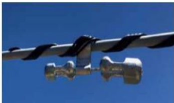
Figure 1: Stockbridge Damper
