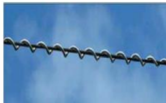
Figure 2: Spiral Damper
