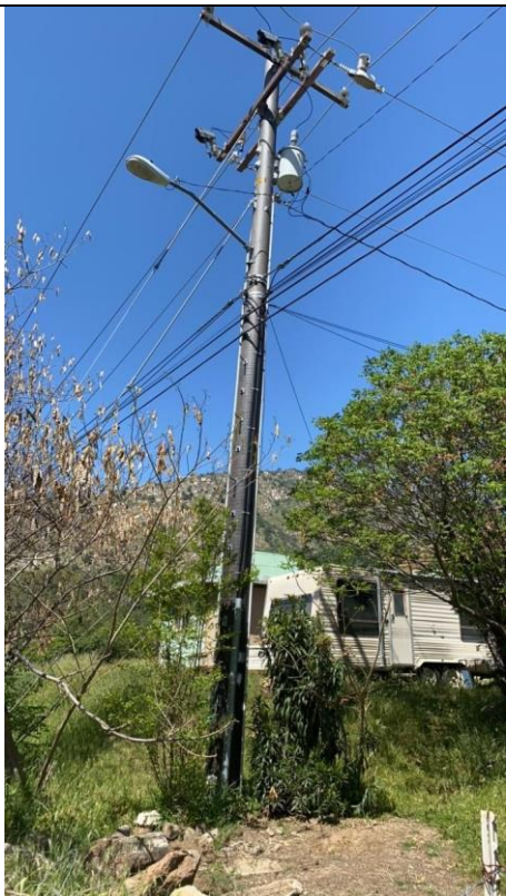
Item6GImg1: Overall pole
