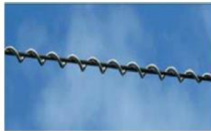
Figure 2: Spiral Damper
