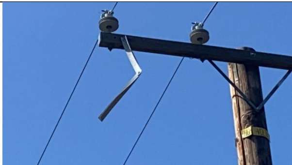
Item11CA2Img1: Wildlife Mitigation device falling off crossarm
