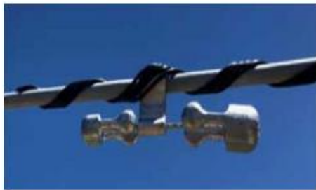
Figure 1: Stockbridge Damper
