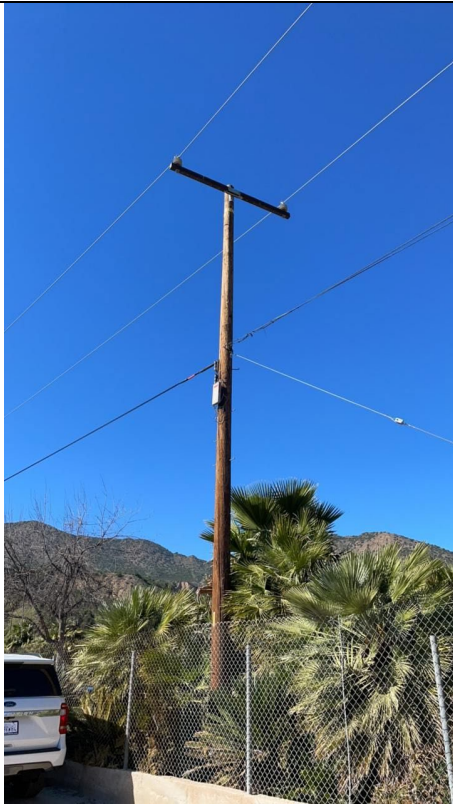
Item2GImg1: Overall pole view
