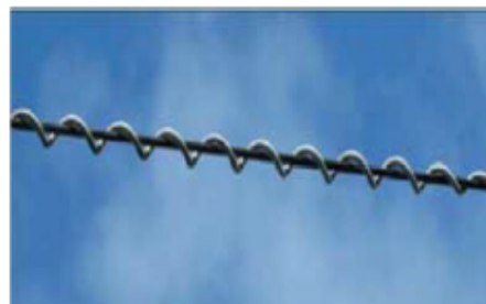
Figure 2: Spiral Damper
