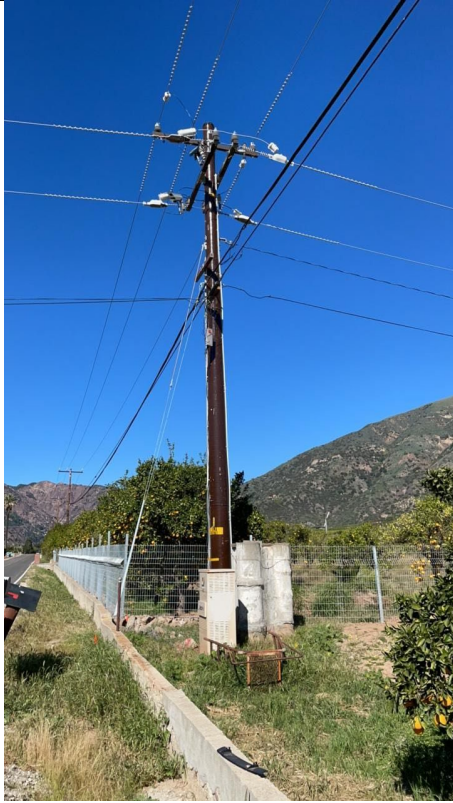
Item3Gimg1: Overall pole view
