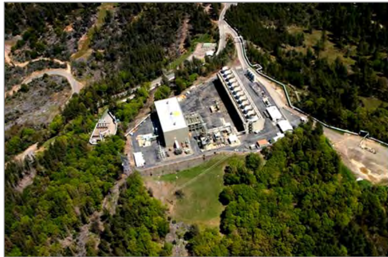
Photo 17-1, Cal Pine Generating Station at the Geysers
