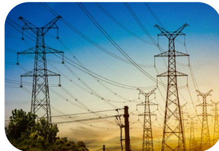
Detailed overhead visual inspections
