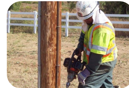
Intrusive pole inspections
