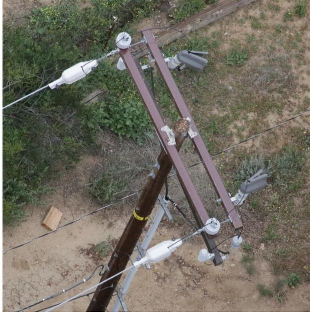
Wildlife Covers: SCE employs wildlife covers on covered conductor systems to mitigate contact risk at exposed connection points. Wildlife covers are installed on dead-ends, terminations, connectors, and equipment bushings. By covering other equipment, contact-from-object faults may be prevented not only with the conductor, but with other energized sources as well. Figure SCE 9-5 shows wildfire covers on a covered conductor system.
