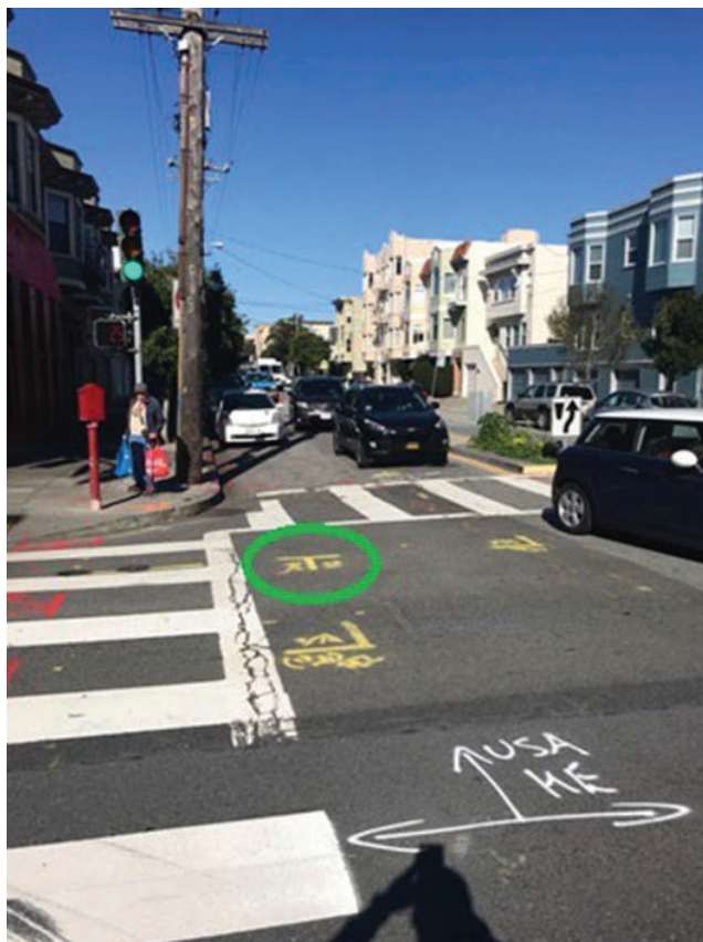
Figure 2: PG&E Locate & Mark Photo, pointing north along Parker Ave. The connection that was struck on February 6 is circled in green. Courtesy NTSB.
