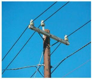
Most of SCE installations on Cross-arm (SCE uses grey to reduce the impact of sun light heating effect, thus increase ampacity)
