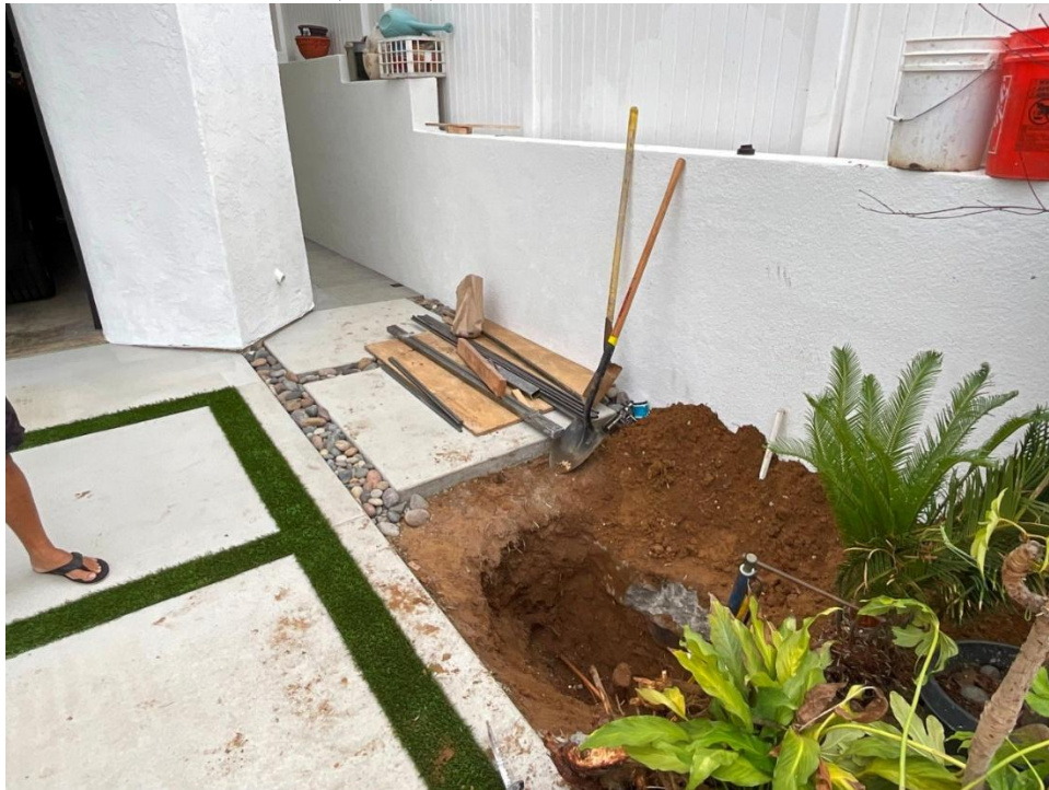
Photo 1: Provided by San Diego Gas and Electric, depicts the excavation area at 2055 Cambridge Avenue, Cardiff, California 92007.
