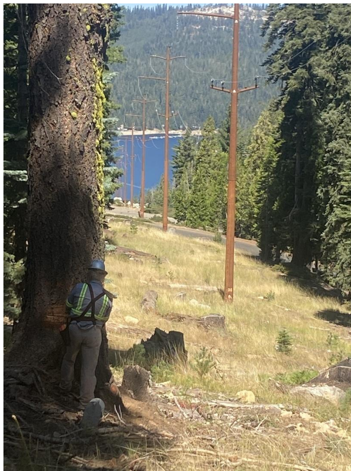
Figure 5 – 2026 Overhead Powerline Corridor
