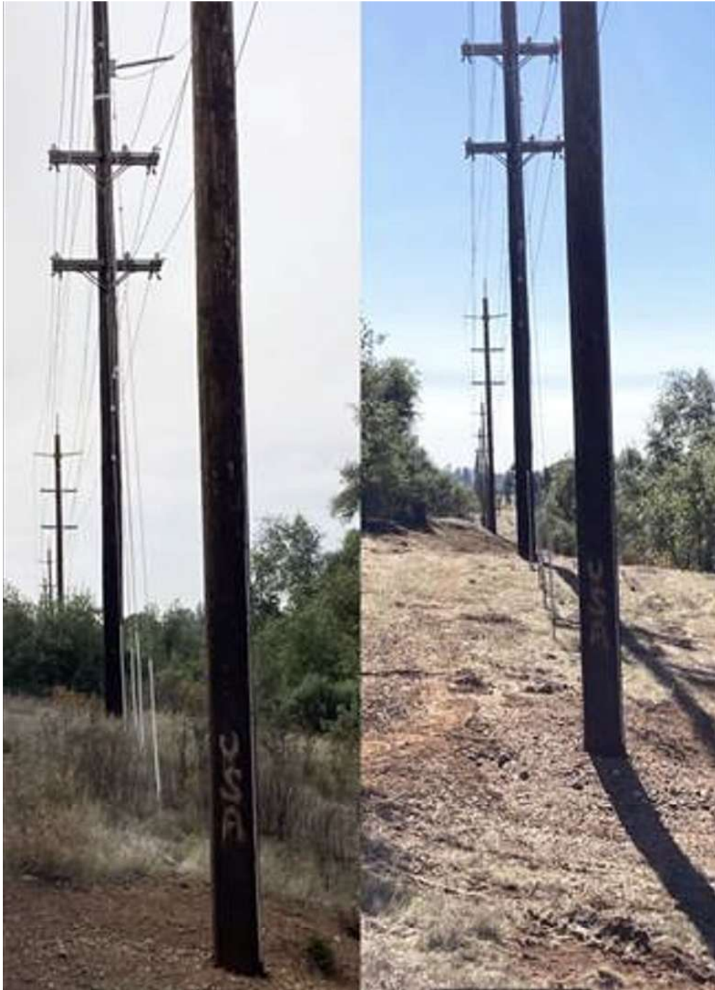
Figure 5-3: Before and After Image of Cleared 115 kV Right of Way. Side-by-side photos of a 115 kV transmission right-of-way before and after vegetation clearance, showing dense vegetation near utility poles on the left and cleared ground around the poles on the right.
