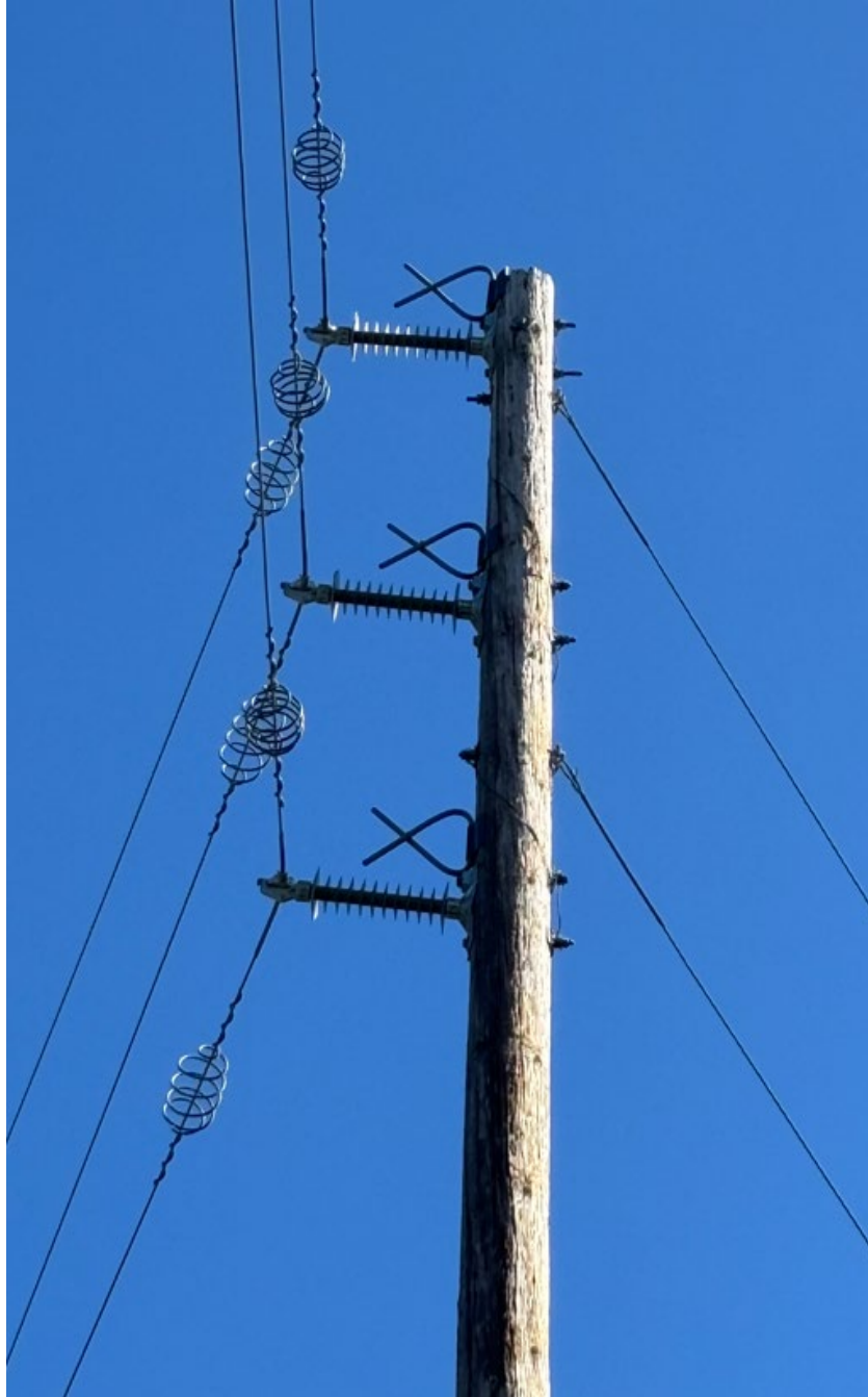
Image 1: Example of Avian Protection, New Hogan Line
