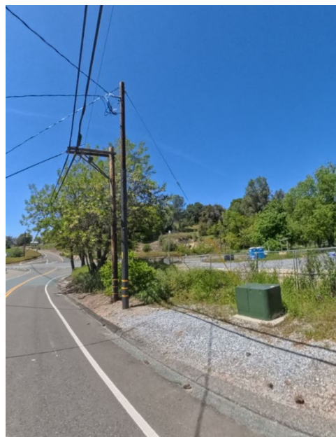
GH ID: [REDACTED] Primary UG to Secondary OH
