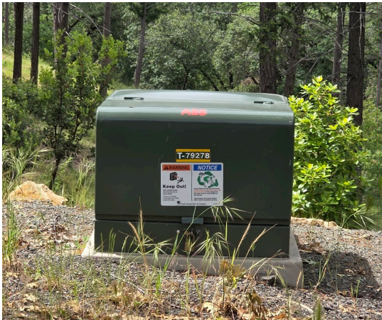
GH ID: [REDACTED] Pad Mount Transformer T-79278
