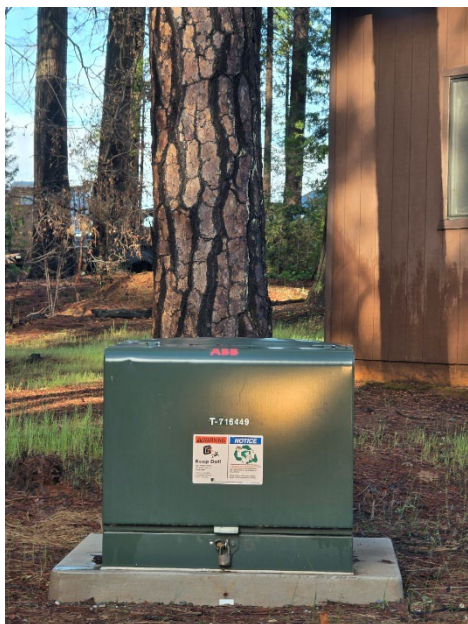
GH ID: [REDACTED] Pad Mount Transformer T- 716449
