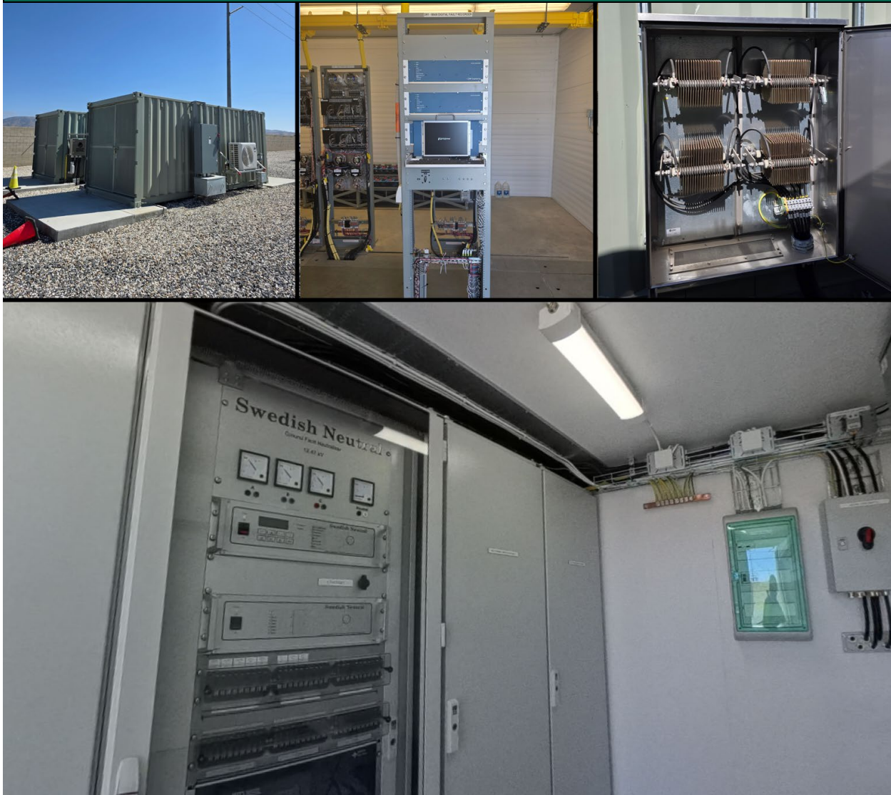
Figure 8: Example GFN Installation
