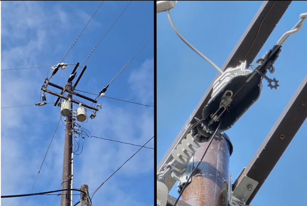
Figure 2: Example Covered Conductor
