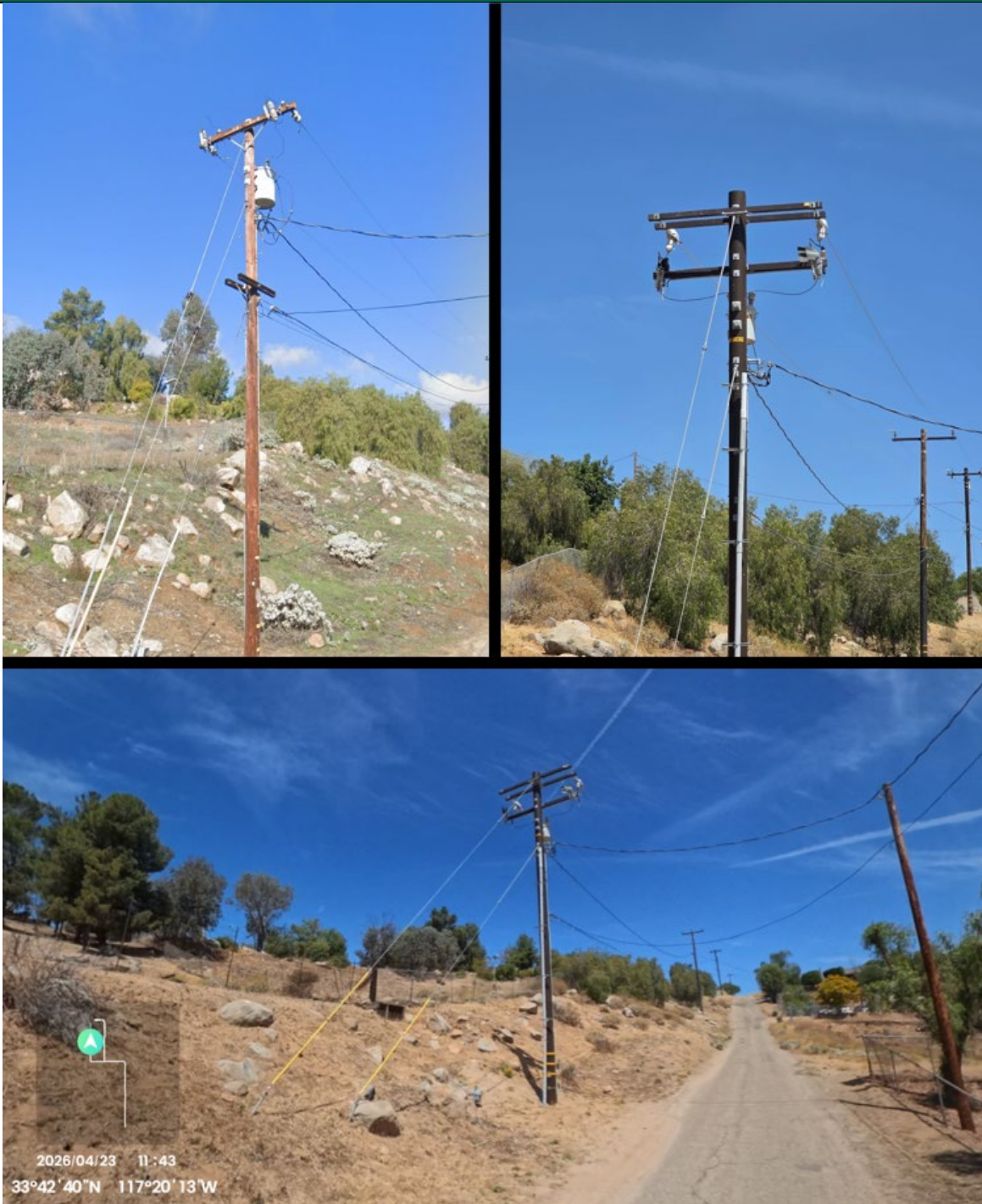
Figure 3: Example Covered Conductor, Pole Replacement
