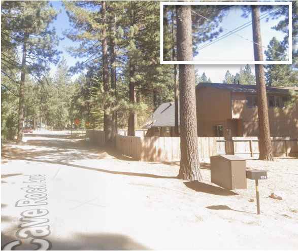
Cave Rock Ave Underground – September 2024 Google Earth Overhead Service 38°56'09.0"N 119°58'41.4"W
