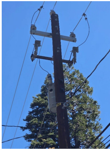
Figure 7: Example of Expulsion Fuse Replacement Field Images
