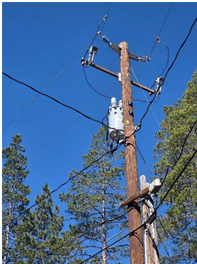
Figure 7: Example of Expulsion Fuse Replacement Field Images
