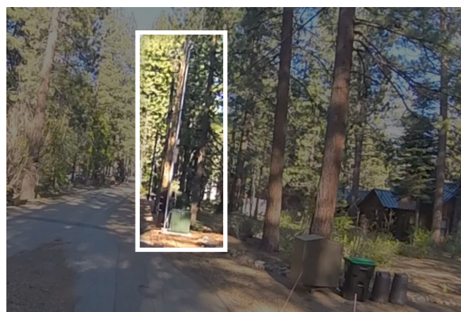
Cave Rock Ave Underground – May 2026 Underground Service 38°56'09.1"N 119°58'45.0"W
