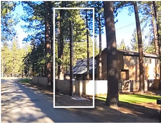
Cave Rock Ave Underground – May 2026 Underground Service 38°56'09.0"N 119°58'41.4"W
