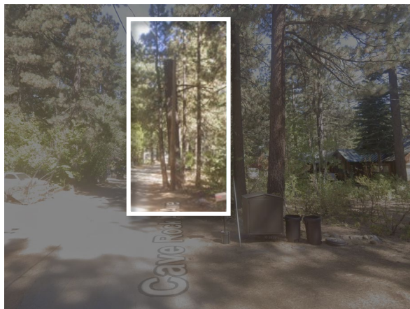
Cave Rock Ave Underground – September 2024 Google Earth Overhead Service 38°56'09.1"N 119°58'45.0"W
