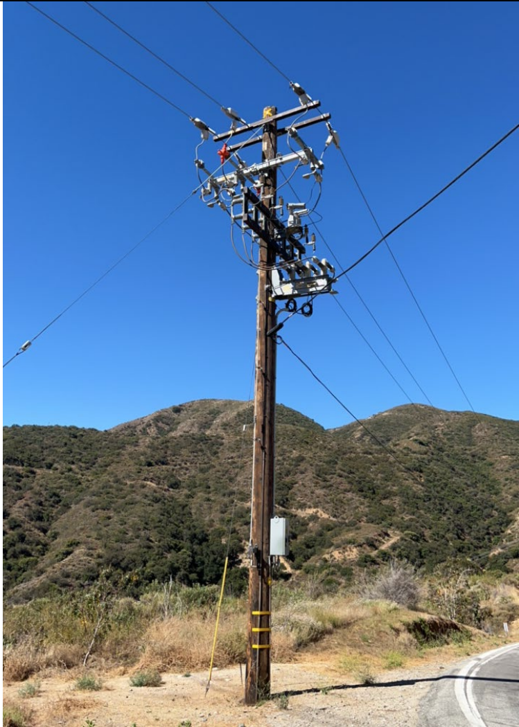
General Image 1: Overall Structure
