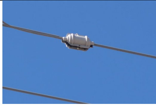
Asset Image 4: View showing unsecured tap cover and exposed bare wire
