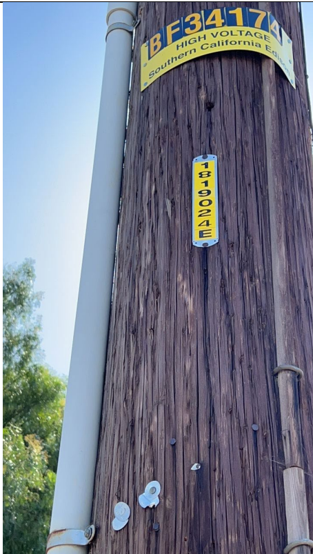
General Image 2: Structure ID
