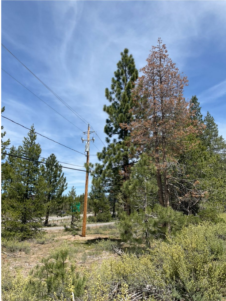
Picture 5: Tree found by Energy Safety (picture from May 20, 2026; removed June 15, 2026)
