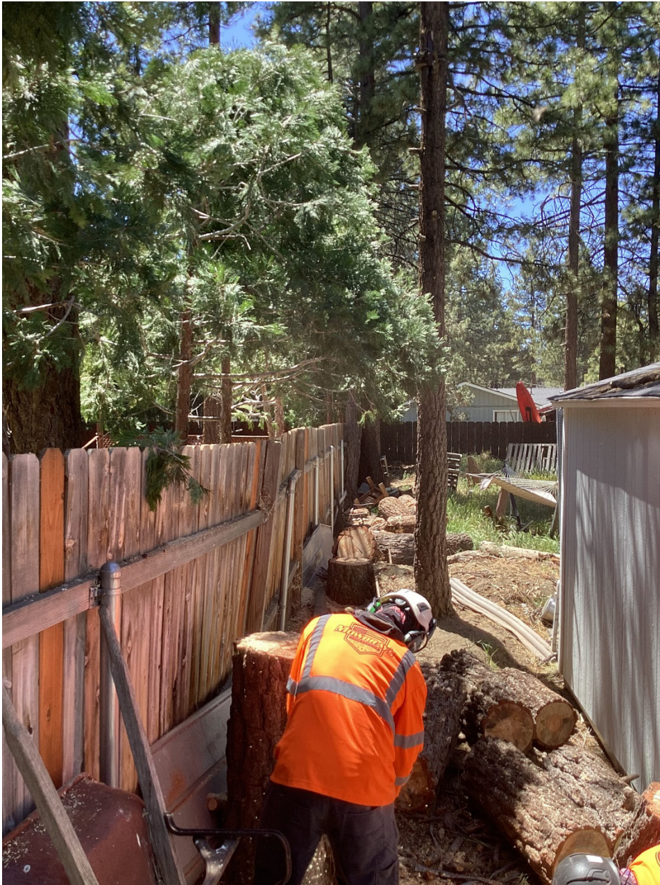
After work was completed.
