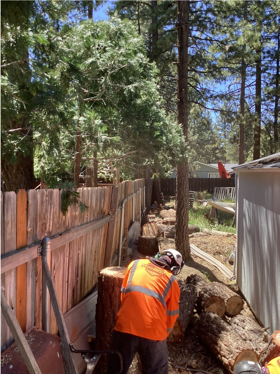
After work was completed.
